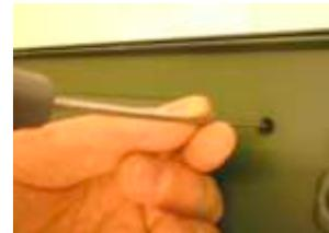
3). Remove Plastic Fixing Rivets.
